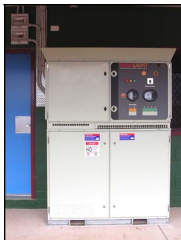
A typical system installed at Corkwood Bore capable of producing 6 kWh/day
